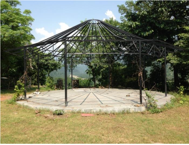
Pavillion for early morning yogas
